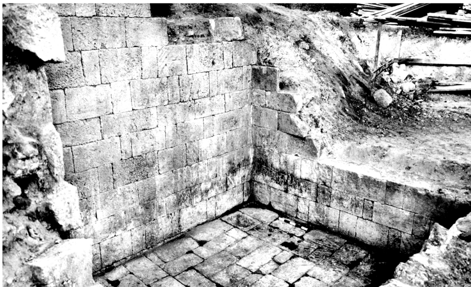
Fig. 3: The ashlar-built structure, looking northeast.
